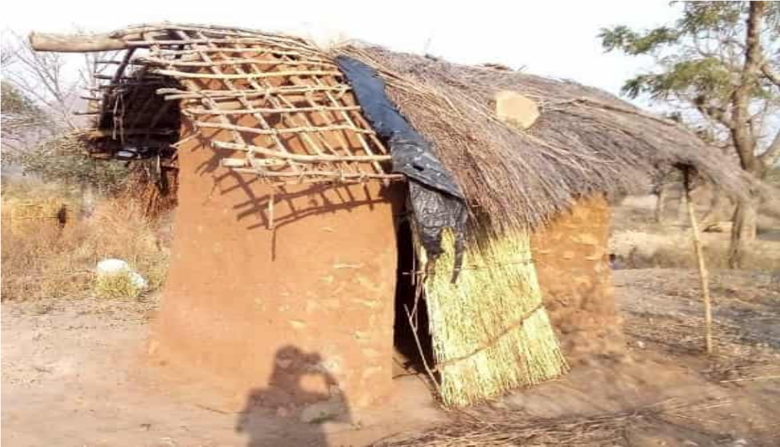
Figure 18: Stone Walls with Mud Mortar, Earth Floor, Grass Thatched House
