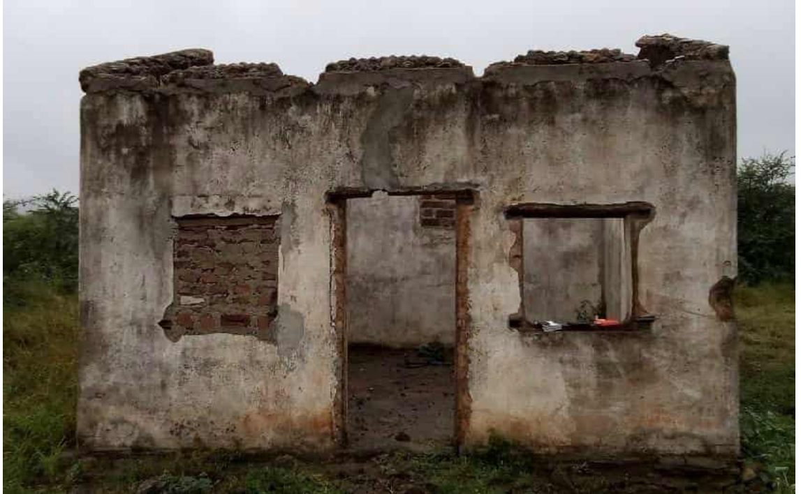
Figure 11: Burnt Bricks, Cement Floor, Plastered, Painted House
