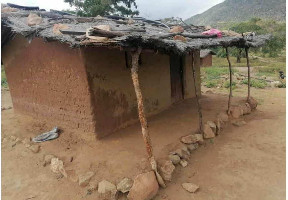
Figure 5: Sundried Brick, Earth Floor, Grass Thatched House
