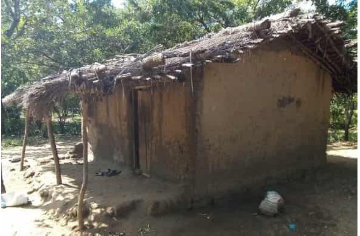
Figure 13: Sundried Brick with Mud Mortar, Earth Floor, Grass Thatched House
