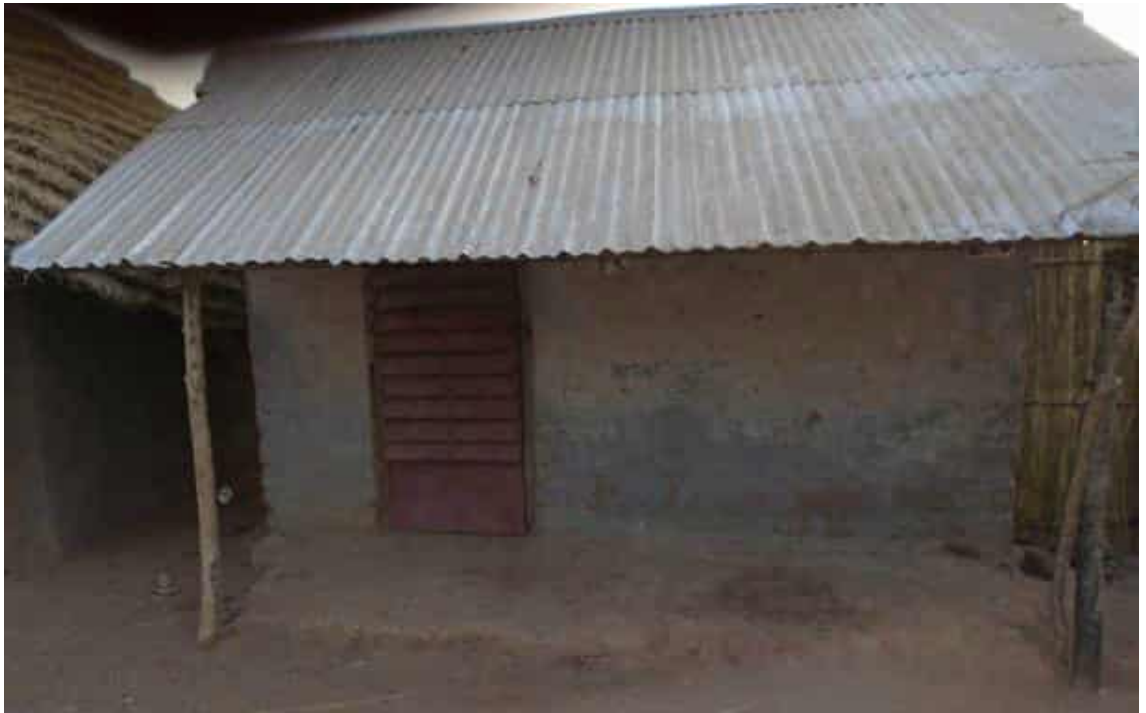
Figure 6: Sundried Brick, Earth Floor and Iron Roof House
