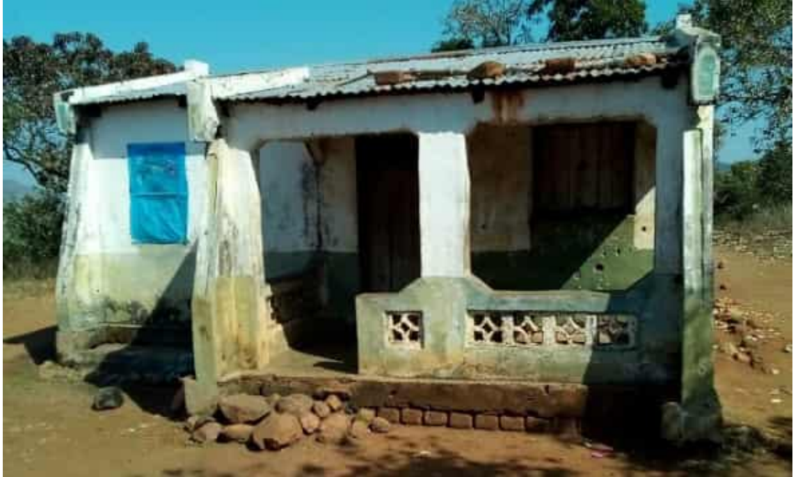
Figure 10: Burnt Bricks, Cement Floor, Plastered, Painted, Corrugated Iron Sheets House
