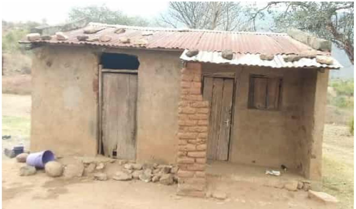
Figure 9: Burnt Bricks, Cement Floor, Plastered, Corrugated Iron Sheets House
